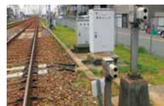
The light signal send and receive units of a level crossing obstacle detection system
