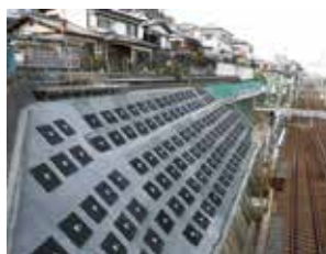
A trackside embankment is strengthened to prevent landslides
