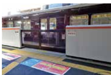
Platform screen doors at Hankyu Juso Station
