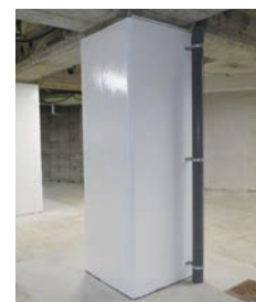
Overbridge support pillar that has been earthquake-proofed
