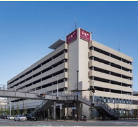
② Hankyu Nishinomiya Gardens Annex
