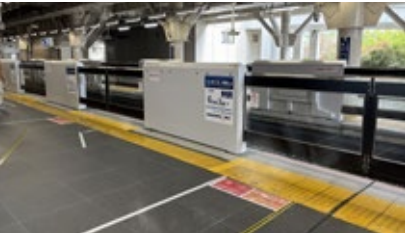
Sliding platform doors at Hankyu Nishinomiya-kitaguchi Station
