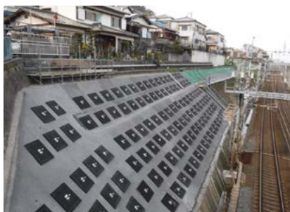
Landslide prevention work beside the track
