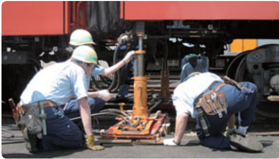
An exercise to return a derailed train to the tracks
