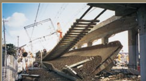
Elevated tracks collapse
