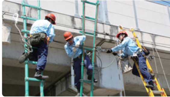
An exercise to repair overhead power cables
