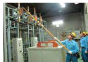
Inspection of substation equipment
