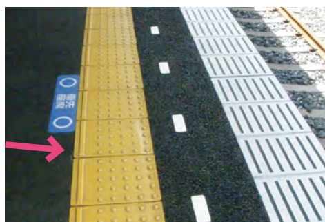
Yellow warning-line tile attached to a platform that conforms to standards established by the Japan Industrial Standards Committee
