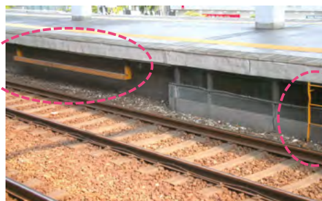
Platform evacuation steps (The dotted line to left shows a bar-type step and the one on the right indicates a ladder-type step)
