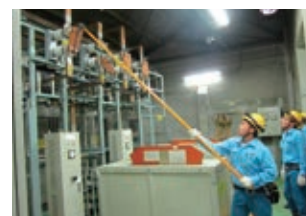
Inspection of substation equipment
