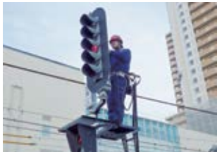
Scheduled inspection of a signal
