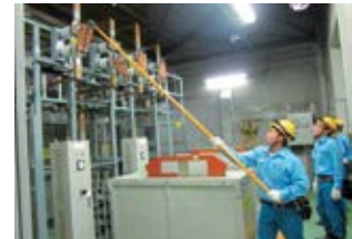
Inspection of substation equipment
