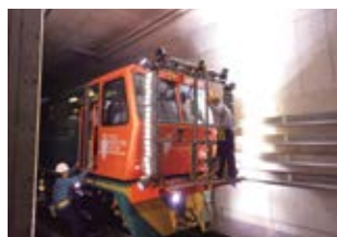
A scheduled inspection of a tunnel
