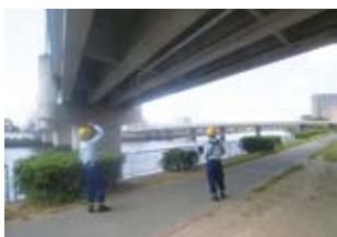
A structure inspection
