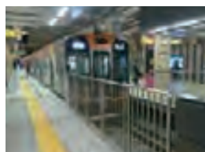
Fixed fencing installed at the head of the platform
