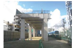
Viaduct construction site
