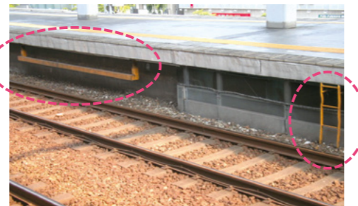
Platform evacuation steps (The dotted line to left shows a bar-type step and the one on the right indicates a ladder-type step)
