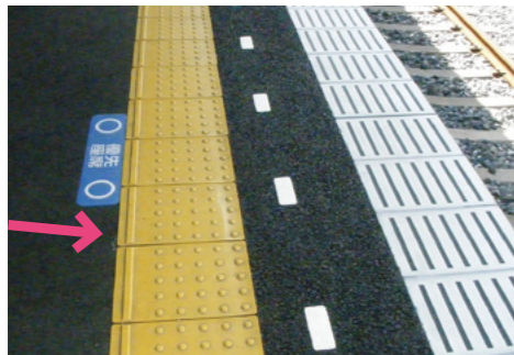
Yellow warning-line tile attached to a platform that conforms to standards established by the Japan Industrial Standards Committee
